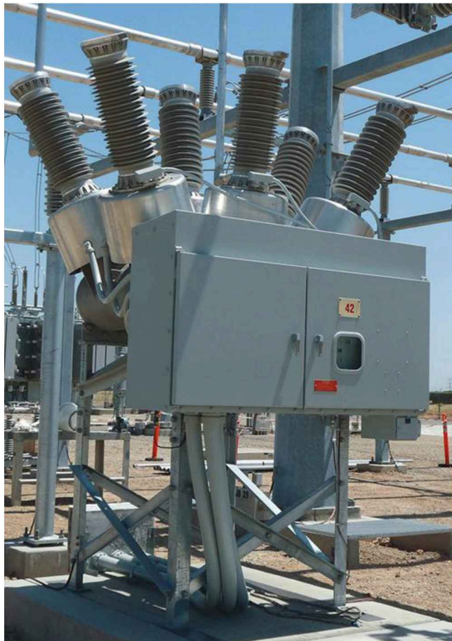
This is during the installation of a 72-kV dry-Air/Vacuum dead tank circuit breaker.
